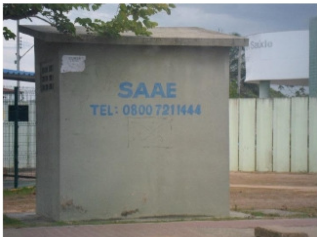
Foto 5.7 – Booster Caique (Fonte: ENGEORPS, 2015)
